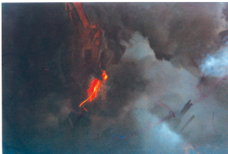
This photograph, taken by Frank Silecchia on September 27, 2001, shows a piece of metal being dug up that is salmon-to-yellow color, indicating temperatures from 845°C (1,550°F) to 1,040°C (1,900°F).
