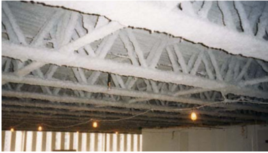
A photograph of WTC trusses with fireproofing.
