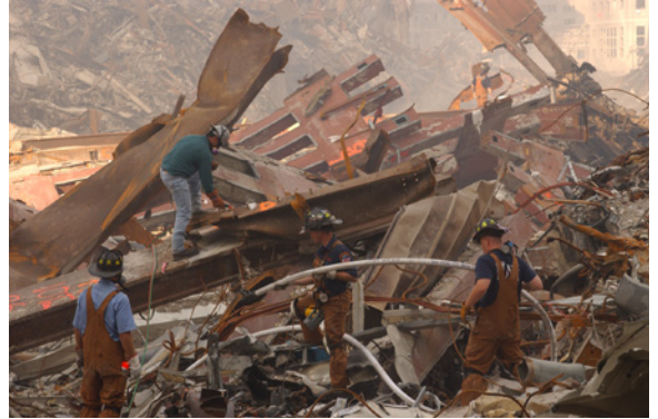
Debris from the dismembered structures of WTC 1 and WTC 2.
