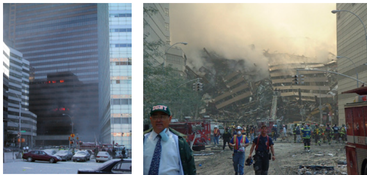
WTC 7 before and after its collapse. Based on NIST's probable collapse sequence, there would be no reason to predict a total collapse until seconds before it occurred.
