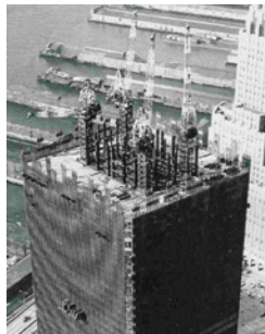
WTC 1 during construction.
